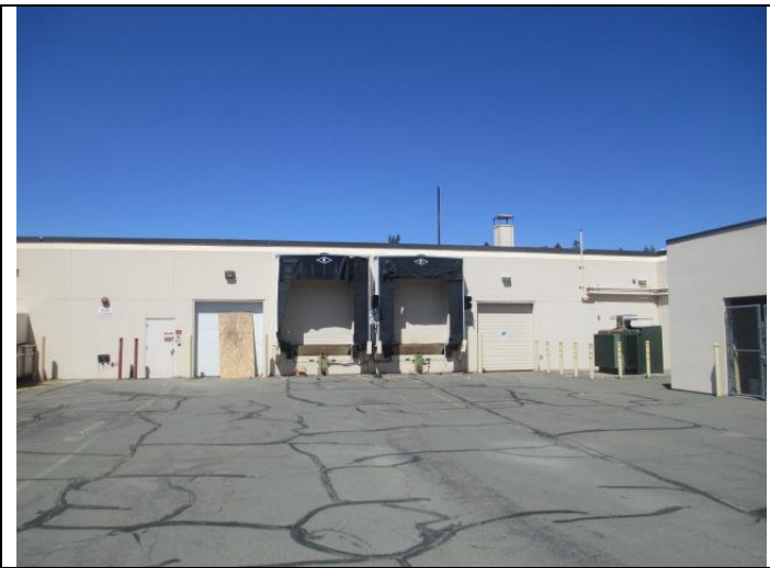
3. View of the south side of the building.
