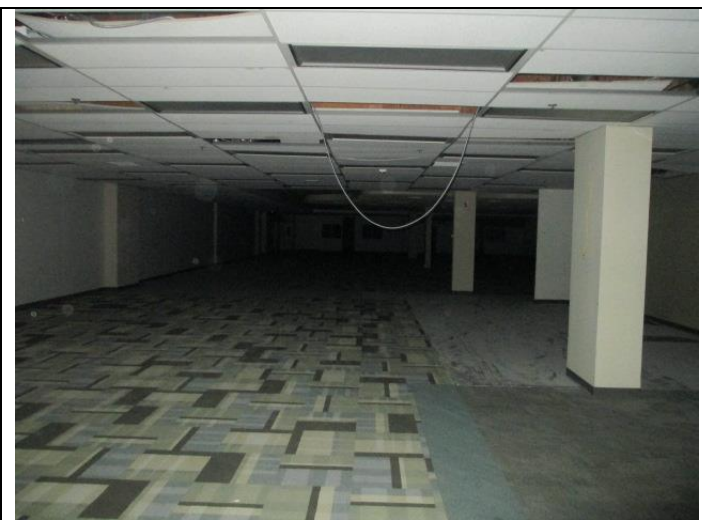
5. View of the former office area.
