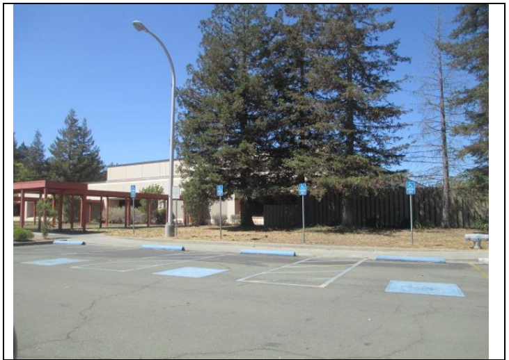
4. View of the west side of the building.
