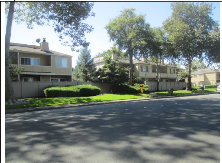
23. View of the adjacent properties south – apartments.
