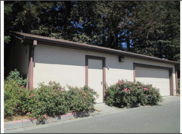
19. View of the irrigation well pump house.
